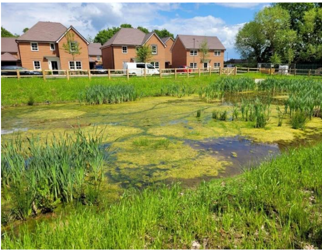
Figure 12 Example of surface water attenuation basin, providing surface water attenuation, water quality, biodiversity and amenity benefit
