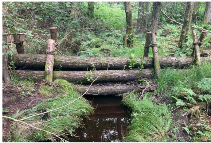
Figure 24 Photo of leaky barrier placed across the watercourse
