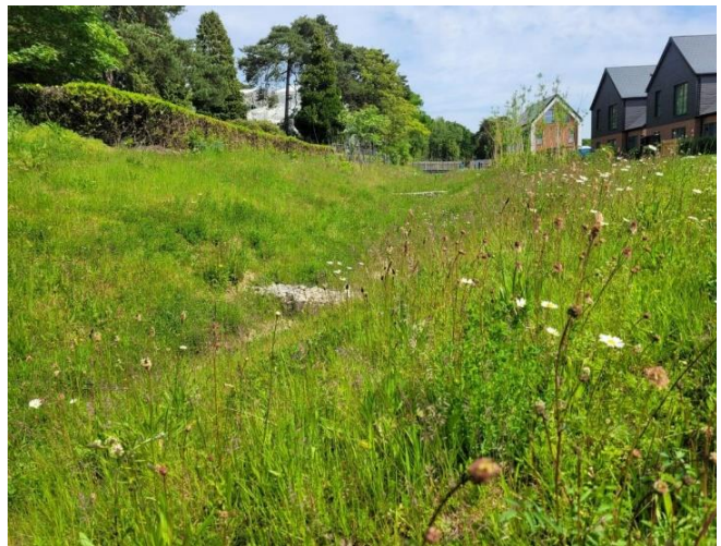
Figure 13 Example of conveyance swale to improve water quality, enable losses of surface water through infiltration and evaporation as well as providing amenity and biodiversity benefits
