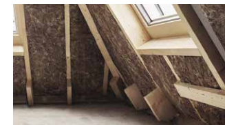
Insulation at rafter level (Source: Knauf insulation)
