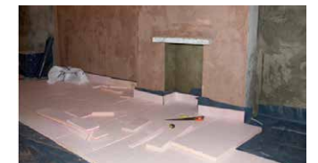
Insulation over a solid floor (Source: rightsurvey)
