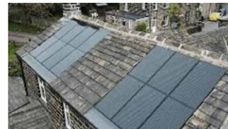
PV installation as tile replacement
