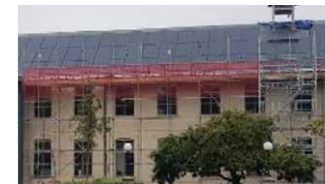
PV installation over tiles
