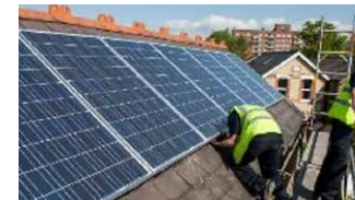
PV installation over the tiles
